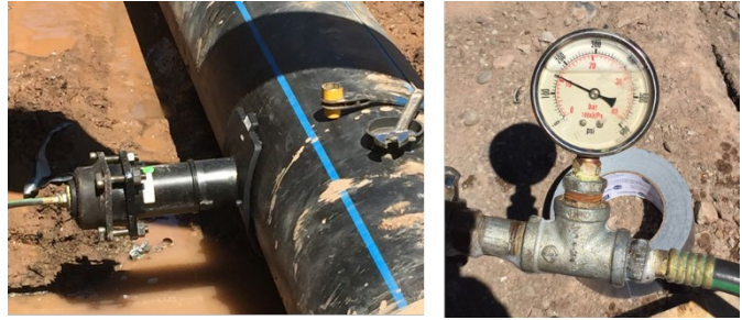
Figure X-p – Pressure Testing
