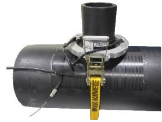
Figure X-n – Place Saddle Over Scraped Surface
